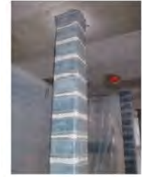
carbon fibres wrapping to increase the shear strength in a column
