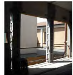
steel encasing for the same purpose
