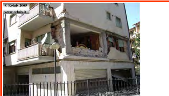
Reinforced concrete building placed in Via XX Settembre – L'Aquila Total and partial ejecting of corner infills at first level.
