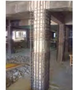
concrete casting to increase shear and flexural strength
